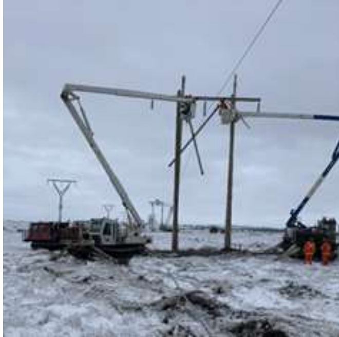
Figure 13: Hydro and Contractor Crews Completing Repairs on TL219
