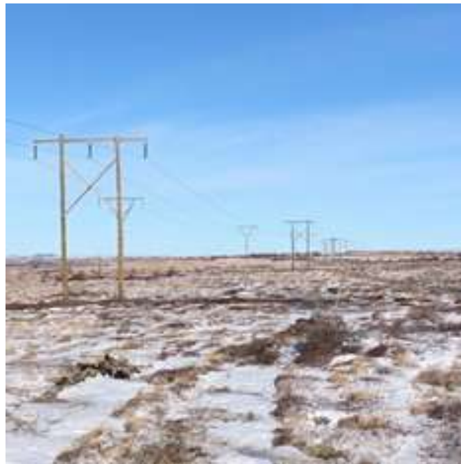
Figure 14: Repairs Complete on TL219
